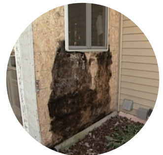
House rot from improper moisture management
